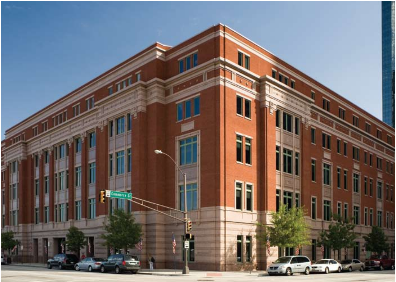
Tarrant County Courthouse
