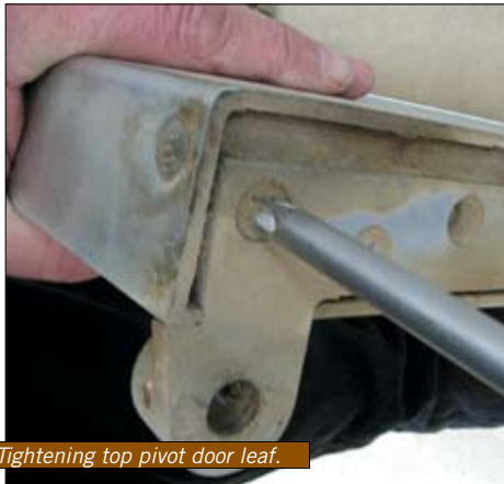
Install spindle arm.
