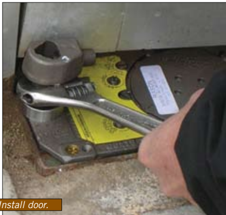
Tightening top pivot door leaf.
