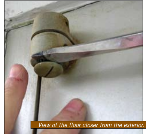
Removing the stud from the top pivot.
