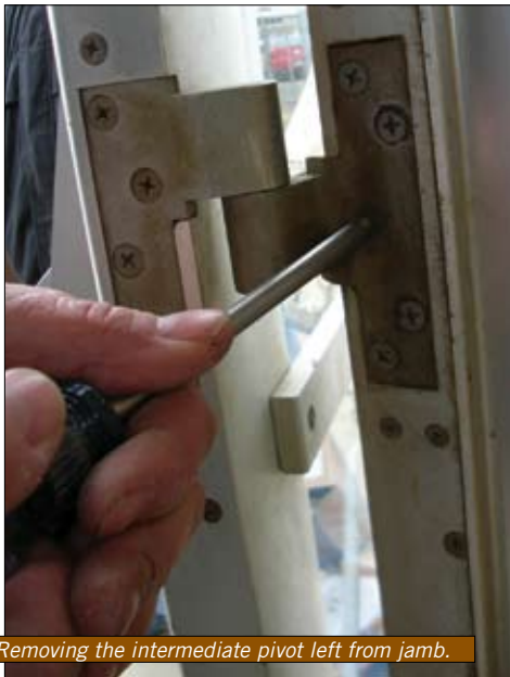
View of the knuckle Note 3/4" bolt.
