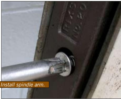
Installing the new floor closer.
